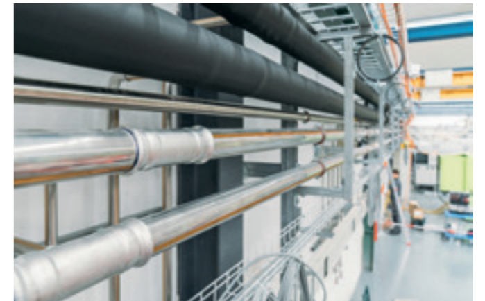
↑ Economical and corrosion-resistant system for cooling lines.
